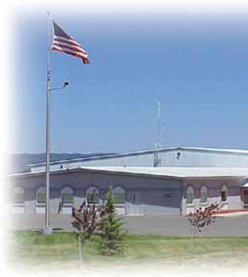
Ashton, Idaho Headquarters Building
